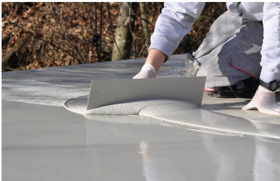
Wecryl 337 - PMMA - Mortier autolissant bicomposant
