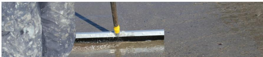
Wecryl 121 A - PMMA - Bouche-pores
